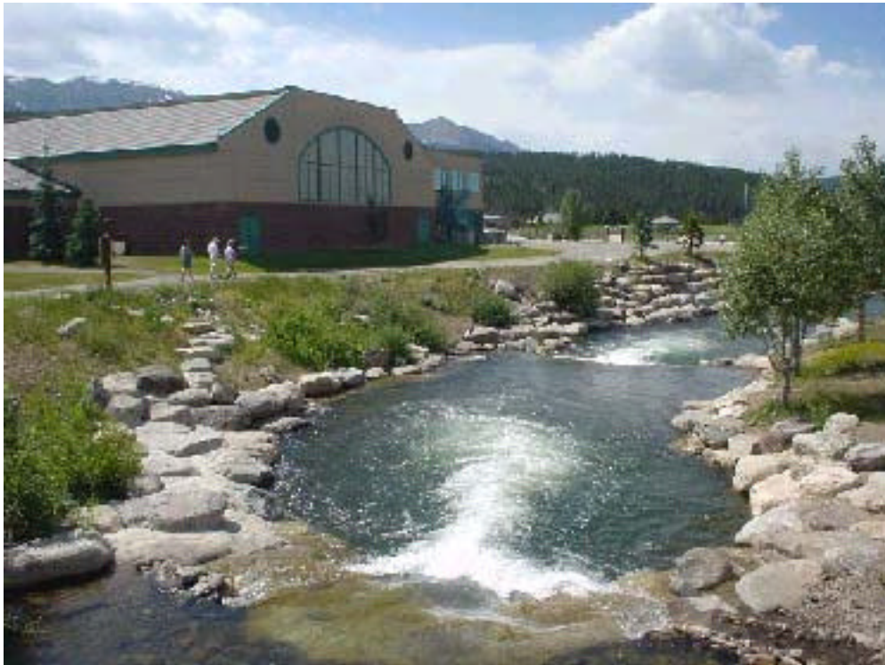
A typical set of drop structures in Breckenridge, Colorado.
